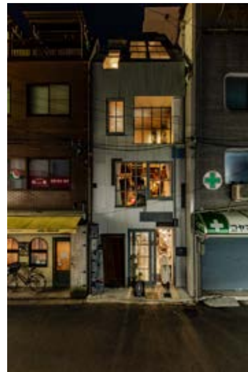
north facade (day to night)
