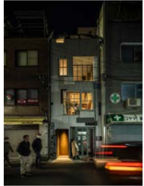
north facade (day to night)
