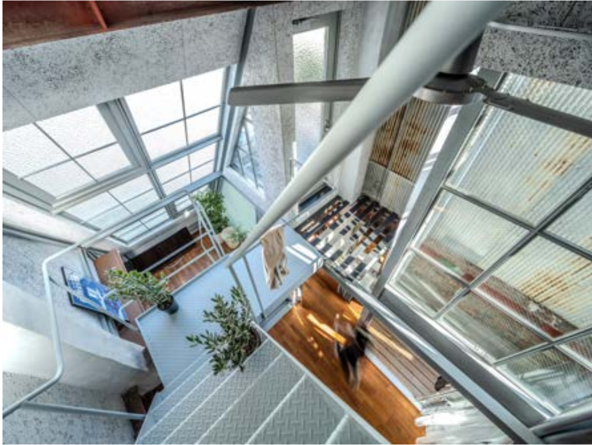
Part of the interior and exterior uses scrap galvalume steel plates from demolition sites.
